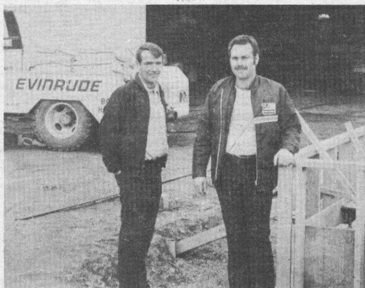
Jack Reynolds and Steve Nelson stand next to the forms for the new building at Ganges.
