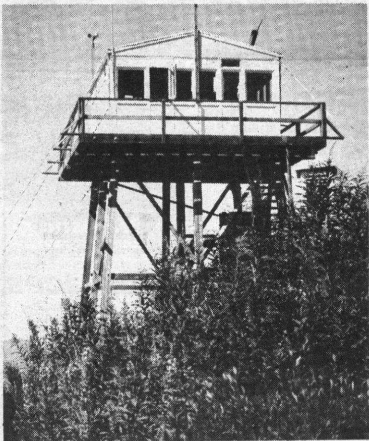
Member of a vanishing species is this Forest Service fire lookout tower on Log Mountain, near Cowichan Lake on Vancouver Island. Today it's used only occasionally as a patrol point. More sophisticated equipment and patrolling aircraft are taking the place of these old structures which at one time were scattered all over B.C.
