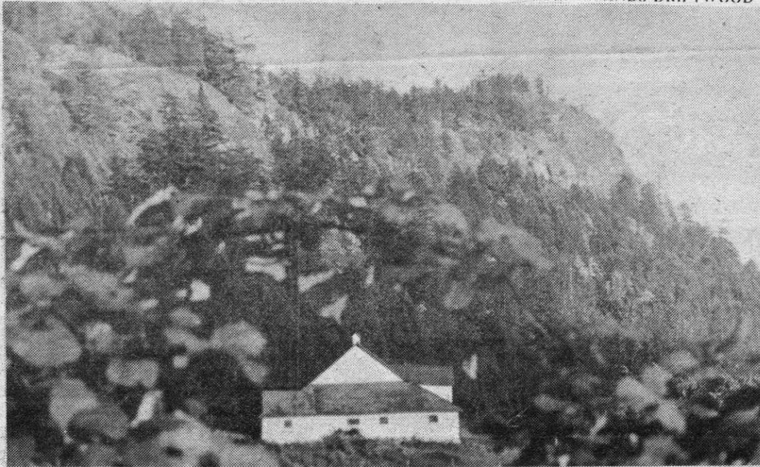
MOUNT PARKE on Mayne Island is the site of a new radar installation being built by K.C. Johnson. Note the old barn, a well known landmark on the island.
