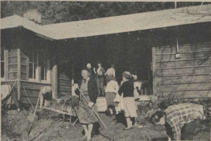
THE WAY IT once was before the recent opening of the new health centre on Mayne Island. Pictured is a work party during a clean-up at
