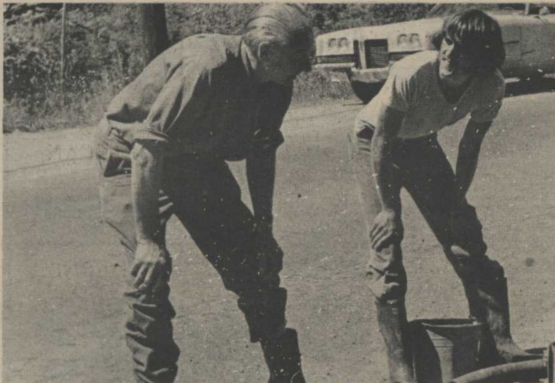
DISCUSSING THE PROGRESS being made to repair a broken water main on the Ganges Hill last week are from left Peter Cartwright and Sandy Blakeway of the North Salt Spring Water District. In the hole below them, fellow worker Mike Larmour was busy fitting a clamp on the main.
