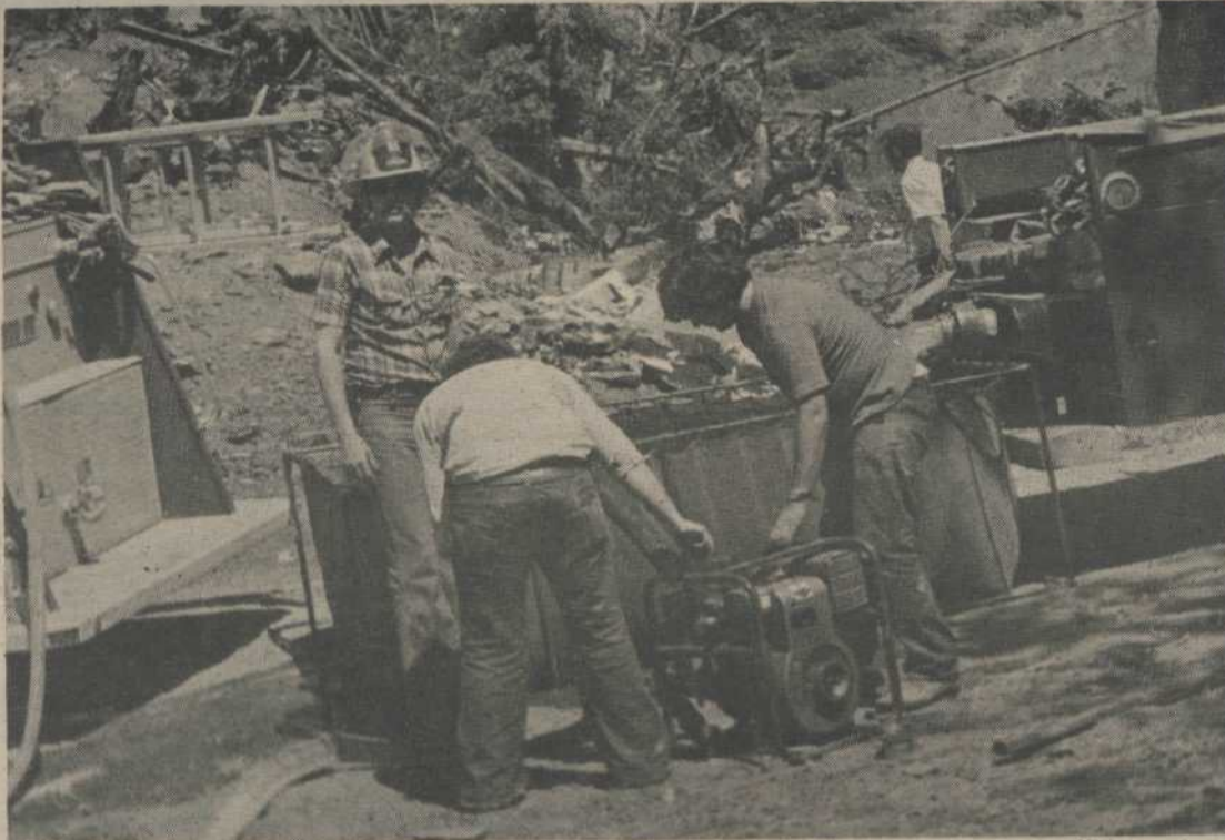
SETTING UP the 1000-gallon porta water tank are firemen, from left, John Andrews (standing), Vern Christensen and Gordon McPhee. In the background is Capt. Lyle Brown. Driftwood Photo
