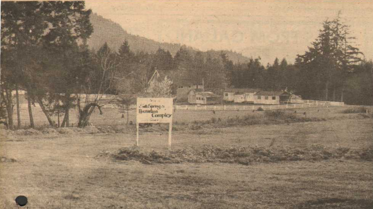
The sign is up at the new recreation complex under construction by Salt Spring Lions. Property at Central has been partially drained and levelled. When the work is finished the field will be lower at his high side and higher on the opposite end.
