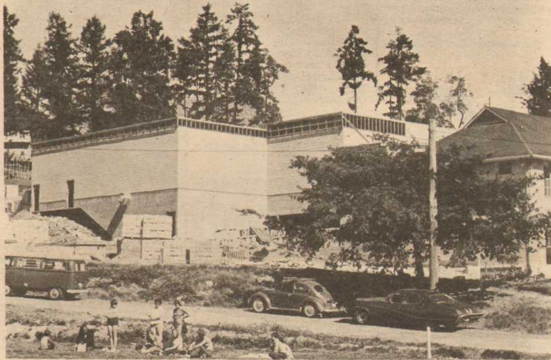
Picture shows the main structure of new extension already built on to the elementary school.
