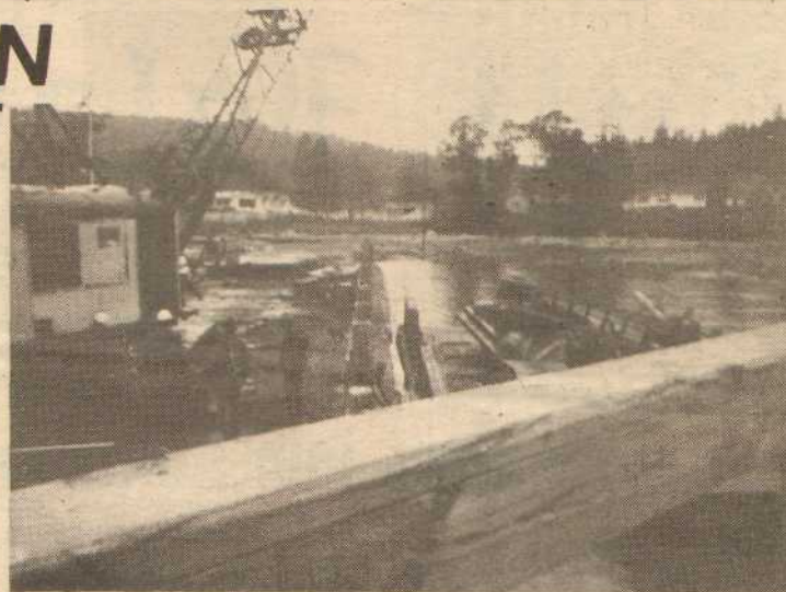
Ferry dock is shipped from one barge to another.
