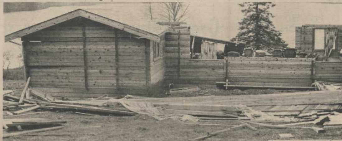
Home of Les Busswood, North Vancouver, is on the shore of St. Mary Lake. The roof was ripped off and dropped in the yard.
