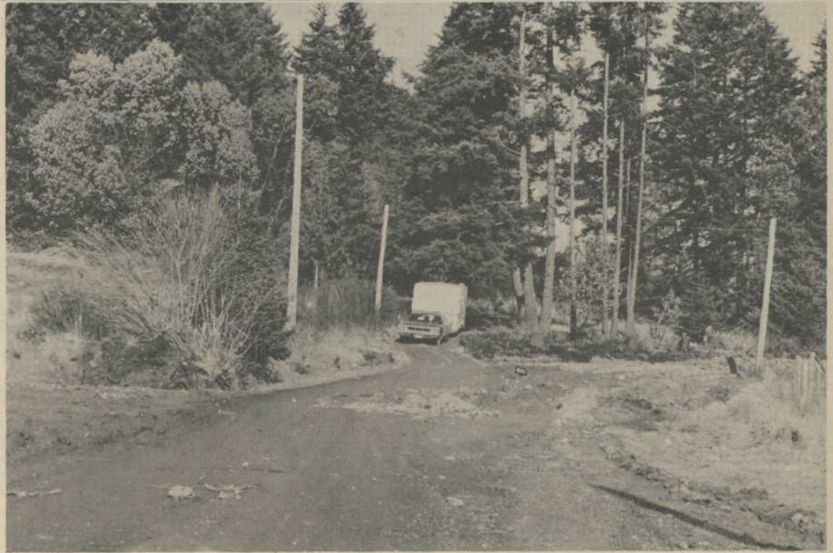
Vehicles on Pender used a temporary by-pass when the road was too wet to accept traffic.
