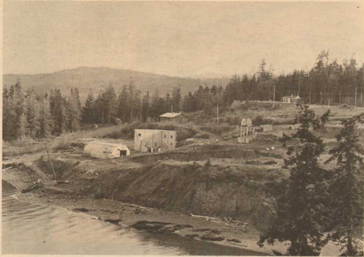
All that remains of the Pozzolan Plant at Welbury Bay
