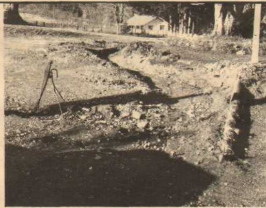
FLOOD WASHES OUT ROAD AT GANGES HOME
