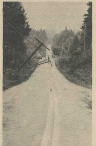
These poles must have been weighed down with water on Friday on Fulford-Ganges Road.
