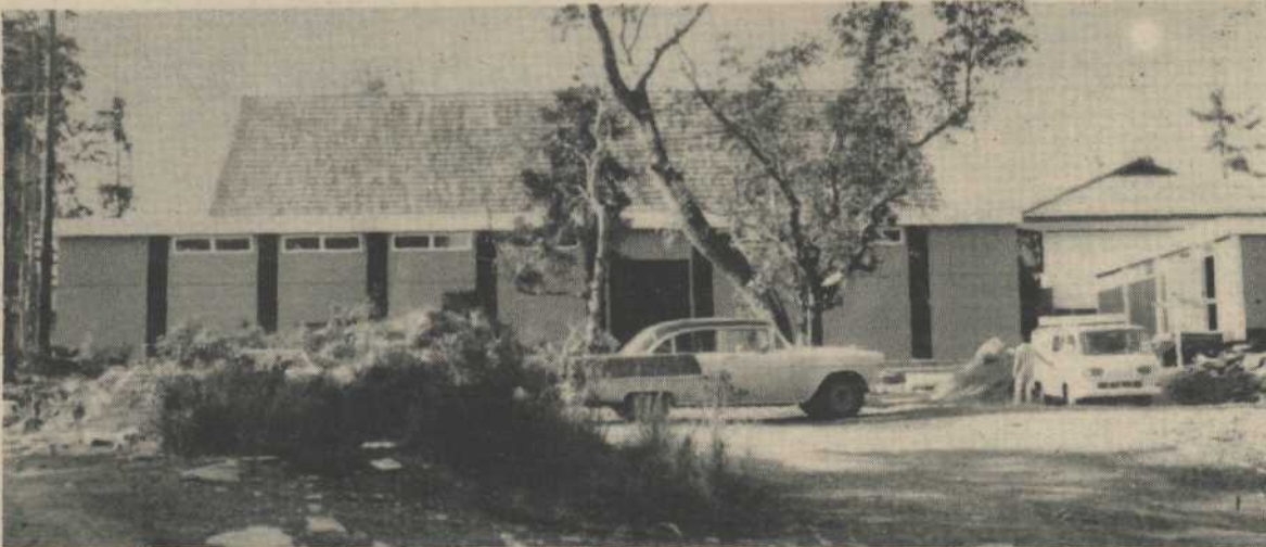
New classroom facilities are nearing completion at Gulf Islands Secondary School.
