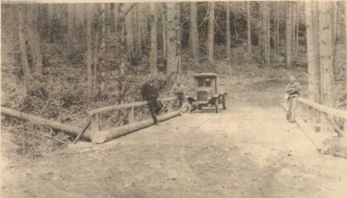
Construction of Cusheon Creek bridge about 1926. Shown are Dick Maxwell, Cliff Wakelin and Roads Foreman Ted Akerman. The Model T was green and was known as the Shamrock.
