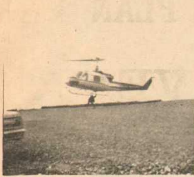
Picking up the pole, the helicopter makes ready.
