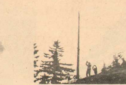
Drops pole gently to B.C. Hydro crew on Mt. Tuam
