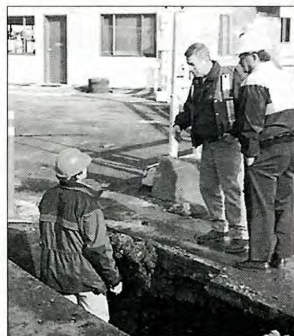
POWER UP —An electrical upgrade to the Harbour Authority facilities at the Coast Guard dock in Ganges came one giant step closer to hook-up last week as Telus, BC Hydro, and Dave's Blasting crews carved and blasted their way across Mout's parking lot to the power source at the entrance to Grace Point Square. When completed, the improvements will not only supply the Coast Guard building and a seaplane wharf with ample power, but will allow the local Harbour Authority to install a marine waste pump-out station on the new breakwater. The Harbour Authority is bearing most of the estimated $20,000 upgrade cost, but thanks to a provincial Beautification Programme, the two utilities are helping out by subsidizing one third of their trenching and line access bill.
