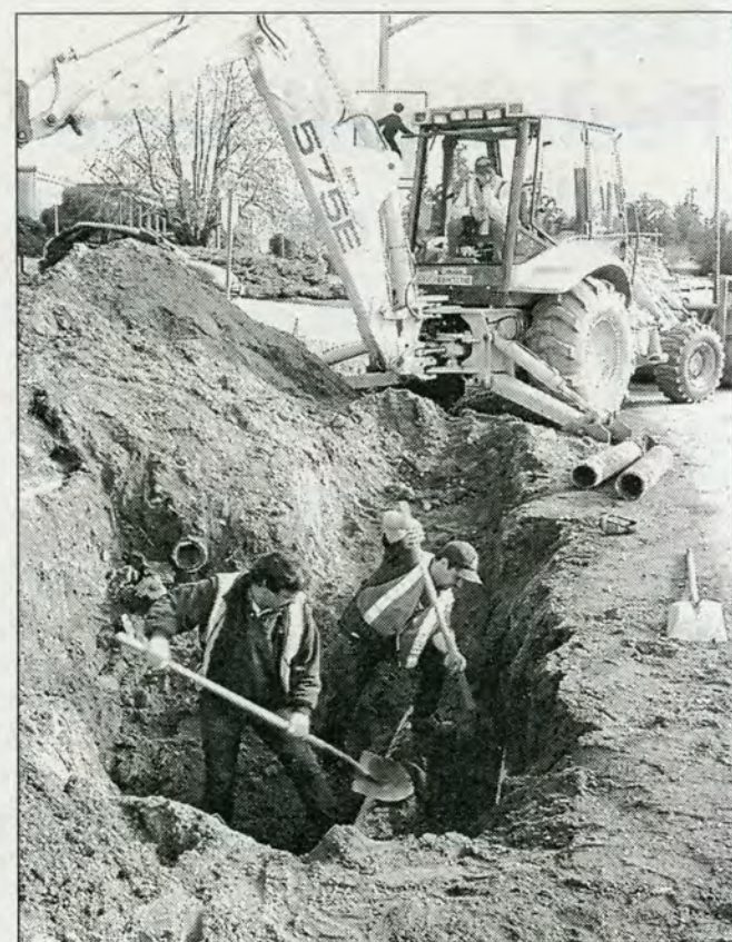
HEAVE HO —Ron Stepaniuk and Ryan Willington are in the trenches digging while backhoe operator Josh Byron looks on. The crew was out at the corner of Lower Ganges and Crofton Roads, installing a new fire hydrant.
