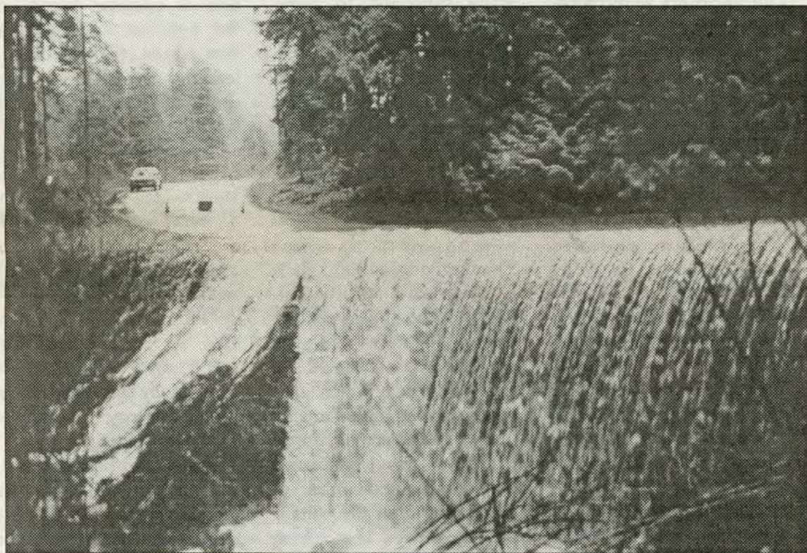
Storm water cascading off a washout on Stewart Road last week Photo courtesy Dave Hogarth.
