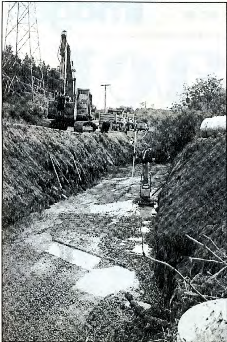
Culvert under construction at corner of Upper Ganges and Long Harbour roads.
