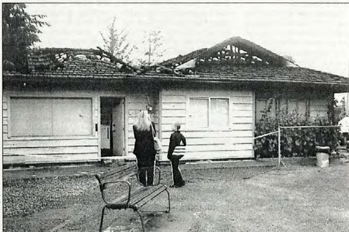
Two hours after being called out, firefighters put the fire out but the blaze left the offices of Parks and Recreation at Portlock Park gutted.
